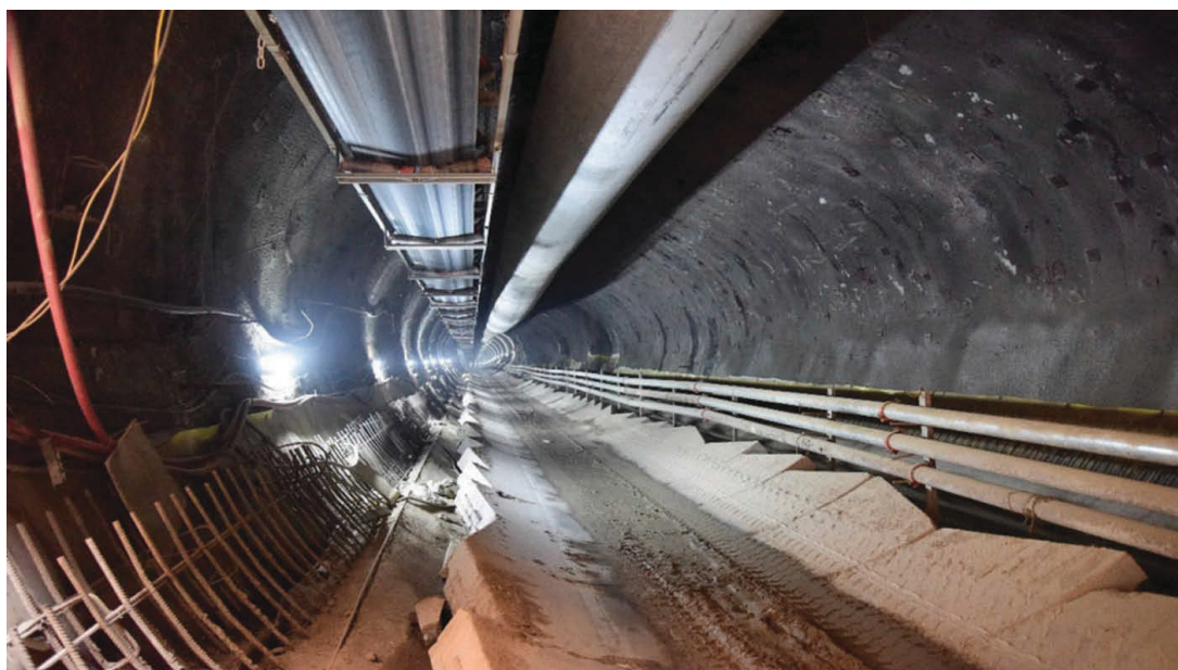
Figure 6. The TBM sliding operation was performed over invert segments through the stations.
