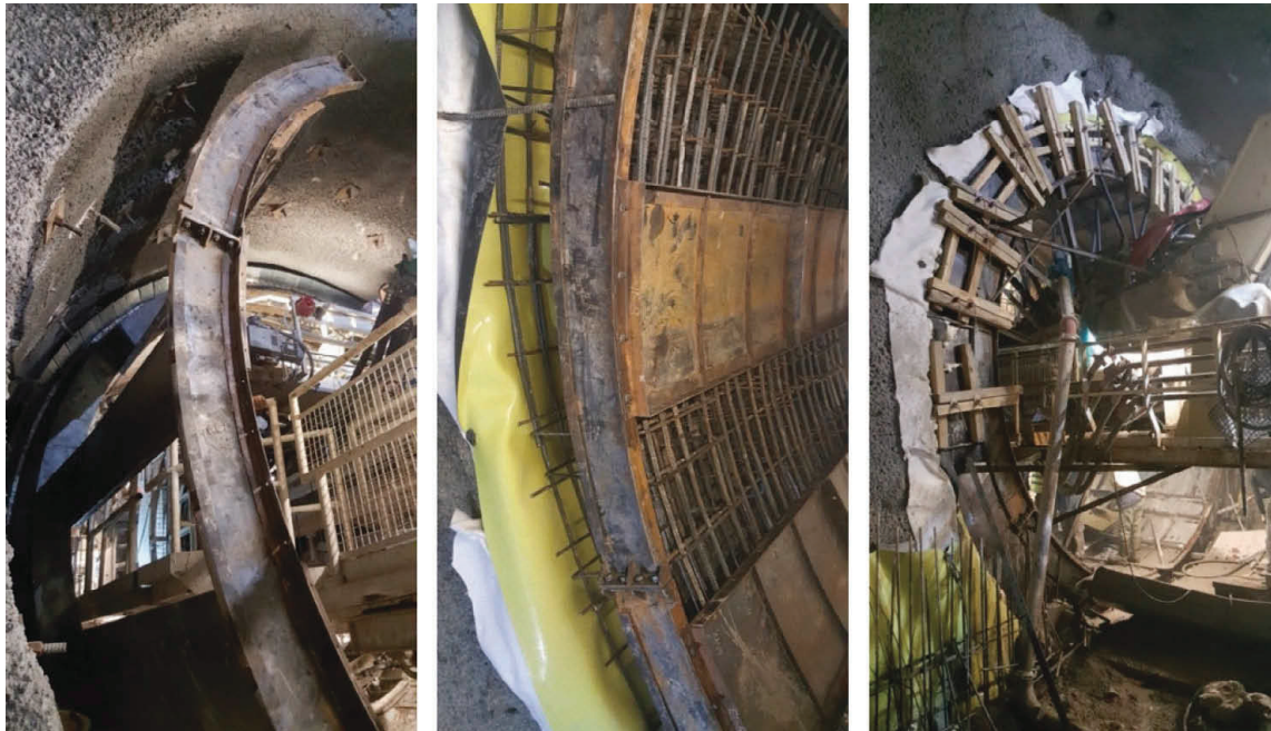
Figure 7. The cast-in-situ TBM thrust ring used at the underground stations.
