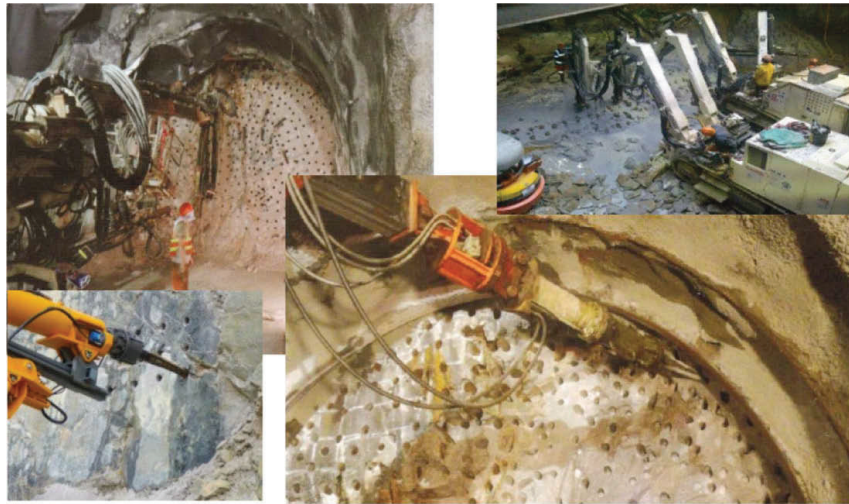
Figure 13. Rock splitting in HK.
