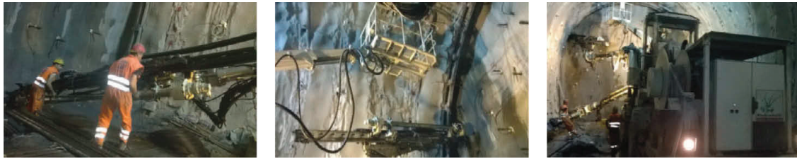
Figure 15. Long holes in faulty zones with 4 booms robotized jumbo and self-drilling bolt carousel.
