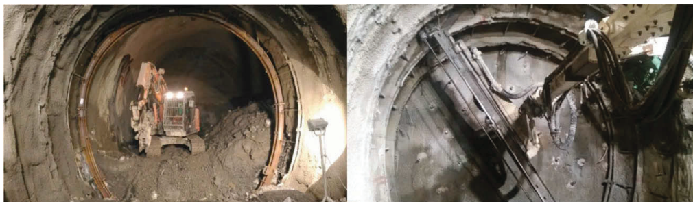
Figure 6. Excavation in a narrow and confined space and self drilling anchors with a 2 boom Robo Jumbo.
