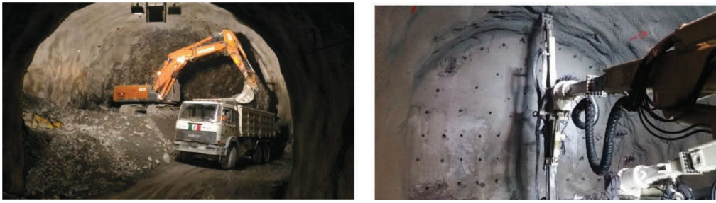
Figure 7. Mucking out in the Exploratory tunnel after the drilling for blast execution.
