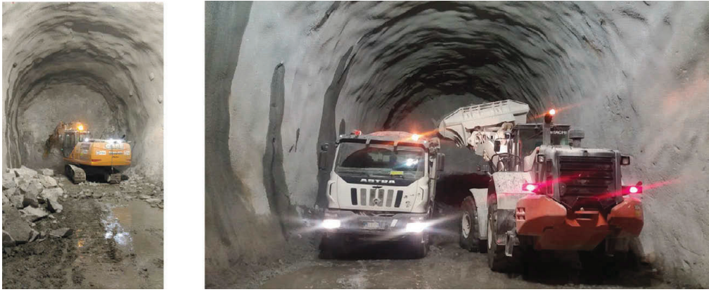
Figure 9. Scaling and muck tipping loading operations.
