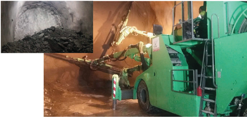
Figure 4. First drilling (blasting) and supporting operations with Robodrill in GA Trens.
