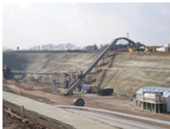
Figure 1. Belt conveyor solution to move material out from a trench.
