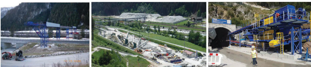
Figure 4. Highway A22 transfer belt to Genauen 2 intermediate waste dump.
