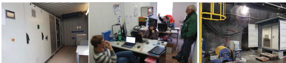
Figure 11. Control rooms and MT's Team in Mules.
