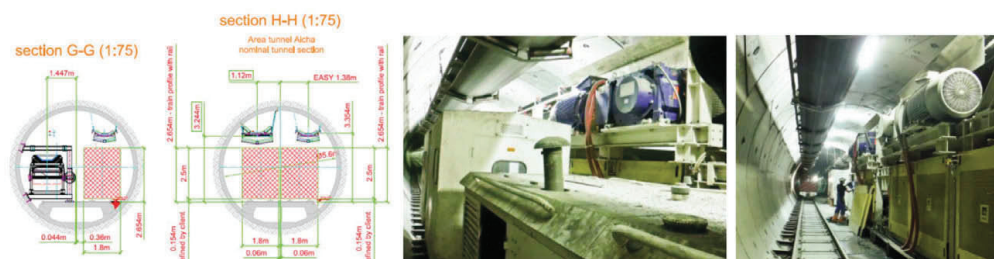
Figure 5. Belts assembly in the Aica-Mules exploratory tunnel with the booster assembly details.
