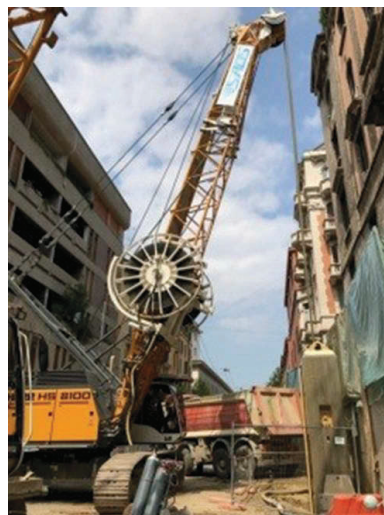
Figure 11. Excavation with slurry grab in down town Milano.
