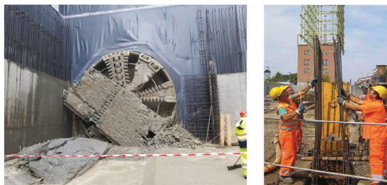
Figure 13. Using the Maplad i-BAR glass fibre reinforced polymer bars.
