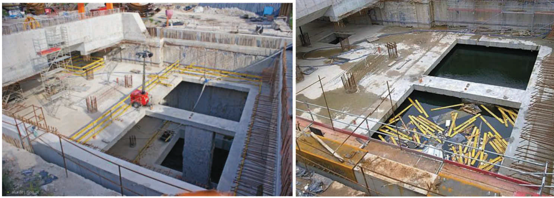
Figure 9. The station before the event and after the intentional flooding.
