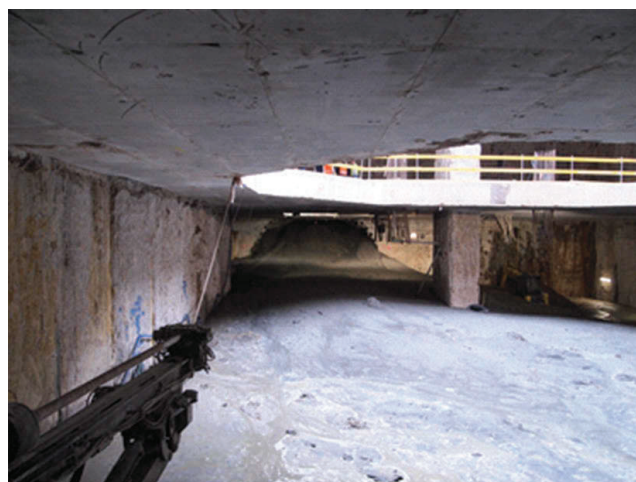
Figure 8. Water, sand and clay inflow from the tunnel.
