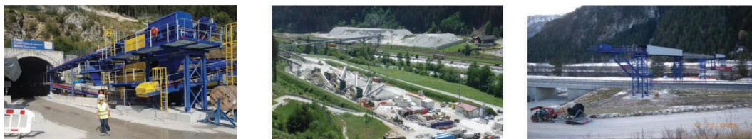
Figure 5. Mules configuration and A22 highway transfer belt to Genauen 2 intermediate waste dump.
