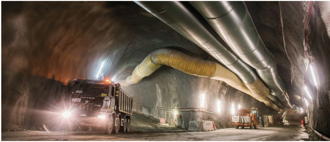
Figure 6. Ventilation ducts in the Mules adit.
